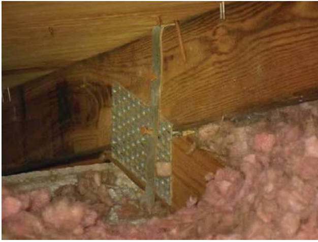
ROOF TO WALL - SINGLE WRAPS
