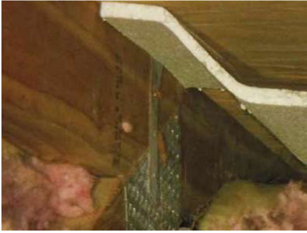
ROOF TO WALL - SINGLE WRAPS
