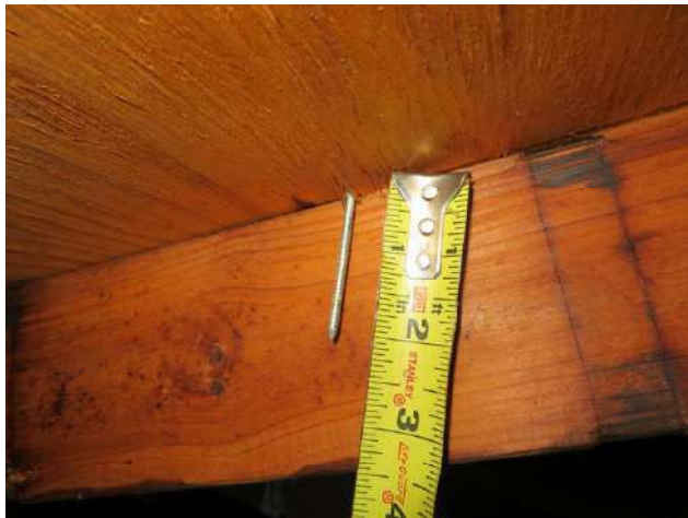
NAIL ATTACHMENT - 8D NAILS
